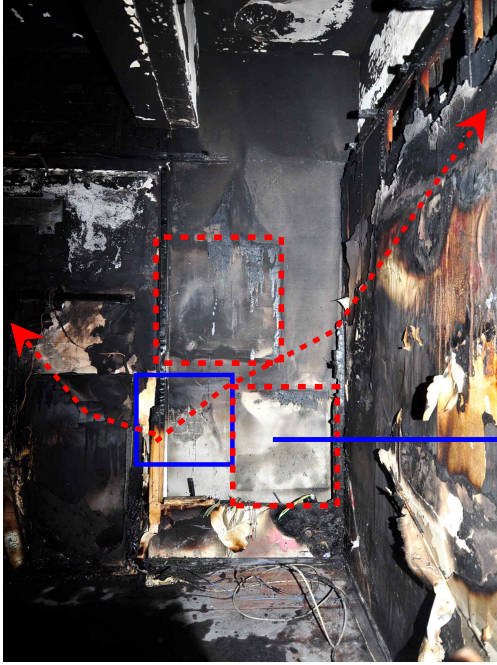
Fig 7. Fire scene around the panel board in the office (The mark is the position of the panel board.)
